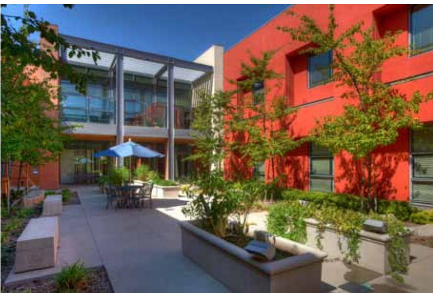
Edgemoor Skilled Nursing Facility
